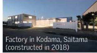
Factory in Kodama, Saitama (constructed in 2018)
